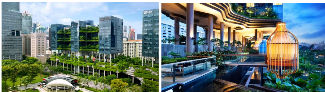
Figures 7 and 8. Parkroyal Collection Pickering Singapore photos. Pan Pacific, Parkroyal Collection and Parkroyal. (n.d.). Retrieved January 18, 2023, from https://www.panpacific.com/en/hotels-and-resorts/pr-collection-pickering/location/gallery.html , 2023.
